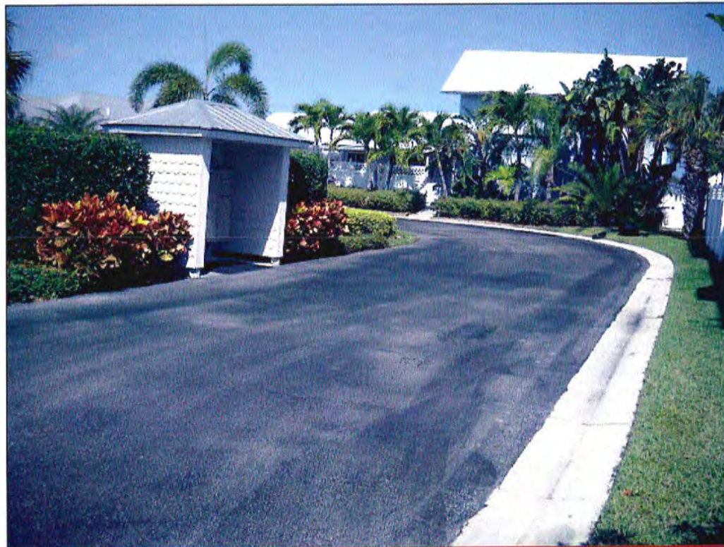
Main Road, Concrete Curbing, & Mailbox Kiosk
