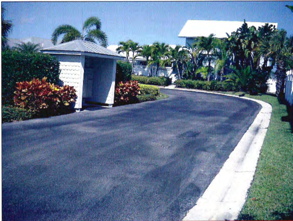
Main Road, Concrete Curbing, & Mailbox Kiosk
